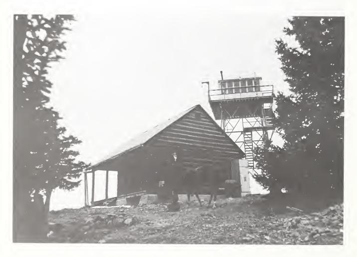
Figure 161. Mogollon Baldy lookout tower, an Aermotor MI-25, and cabin (built in 1923) on the Gila.
